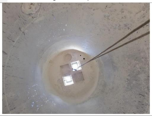
Photo No: 02 Pre-Clean: View showing accumulated deposits to the internal wall surfaces.
